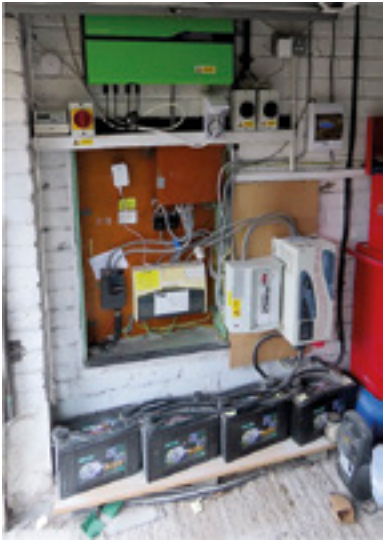
Fig 14: Domestic PV Power conversion and battery back up
