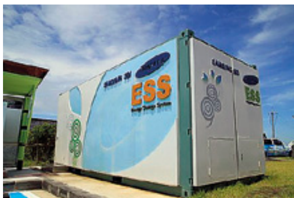
Above and below: Samsung SDI containerised lithium-ion energy storage systems, as to be used by S&C Electric at a trial in Leighton Buzzard, UK.
