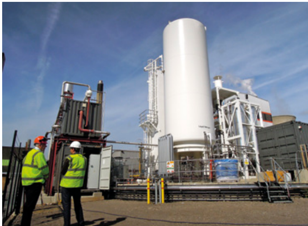
Highview's 300kW cryogenic energy storage pilot plant in Slough, UK.
